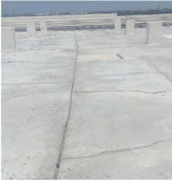
Cracking
